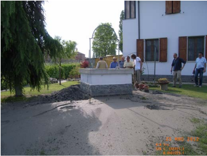
Fig. 30. Ejection of sand from water well (S. Carlo).
