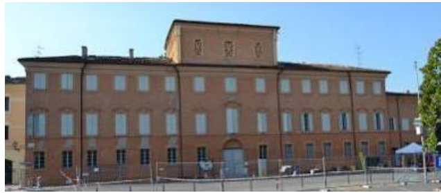
Palazzo Sartoretti – the Town Hall (the main façade)
