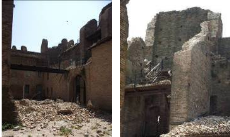
The medieval “Rocca” (collapse events)
